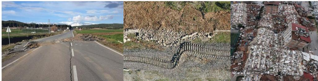
Figure 4. During the 06 February 2023 Pazarcık, Kahramanmaraş, Turkey earthquake, the 3 m offset on the highway and railway and the damage to the buildings can be seen in the region.
